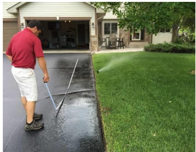
IRRIGATION SYSTEM THAT NEEDS TO BE ADJUSTED SO WATER IS NOT WASTED
