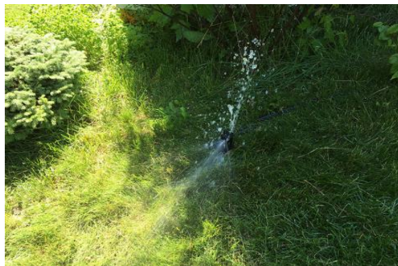
REPLACE BROKEN AND LEAKING SPRINKLERS
